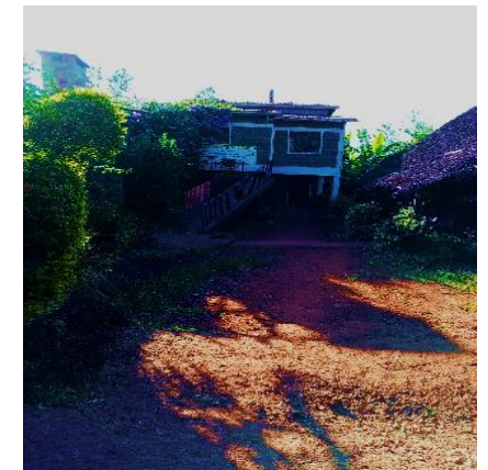
Computer Centre; Meeting Room
